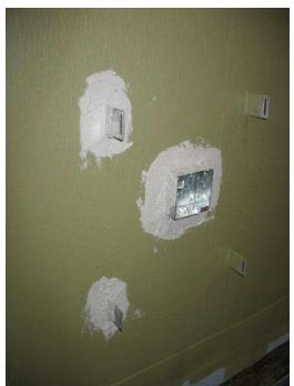
Figure E-10 – Application of LATAPOXY Waterproof Flashing Mortar around Brick Ties and Square Electrical Junction Box / Adjacent Brick Ties Sealed with LATICRETE Air & Water Barrier
