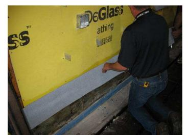
Figure E-3 – Application of LATICRETE Flexible Sealing Tape along Concrete Foundation Interface
