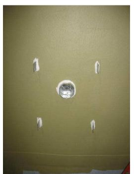
Figure E-11 – Application of MVIS Silicone Sealant around Brick Ties and Hexagonal Electrical Junction Box
