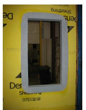
Figure E-1 – Application of LATICRETE Flexible Sealing Tape around Window Rough Opening
