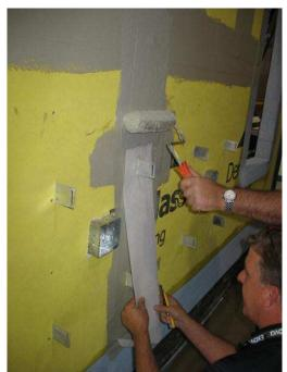
Figure E-5 – Application of LATICRETE Waterproof/Anti-Fracture Fabric along Sheathing Joint / Brick Ties
